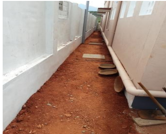
South side Compound wall
