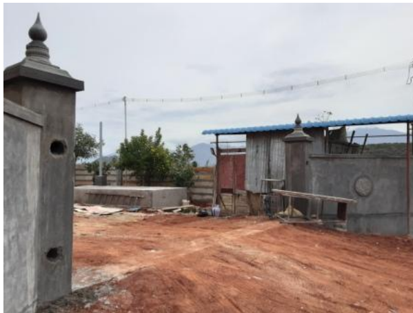
North side Compound wall
